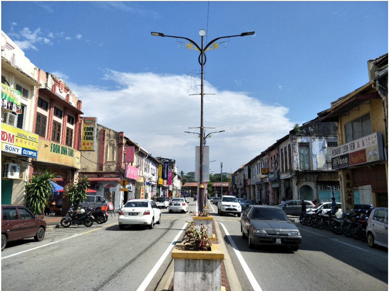
Figure 1: The multi-cultural living heritages of shop houses on Jalan Besar, Tanjong Malim.
